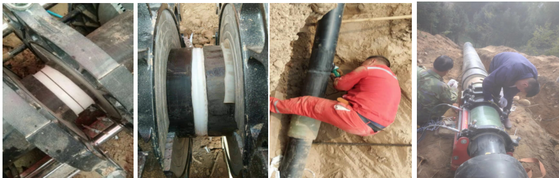
Non-metallic sleeve on-site connection
